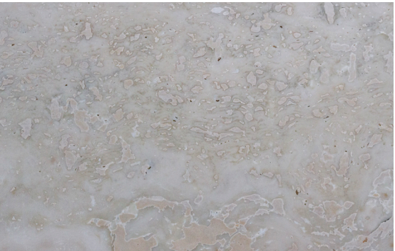
stuccatura mastice (dettaglio) - putty grouting (detail)
